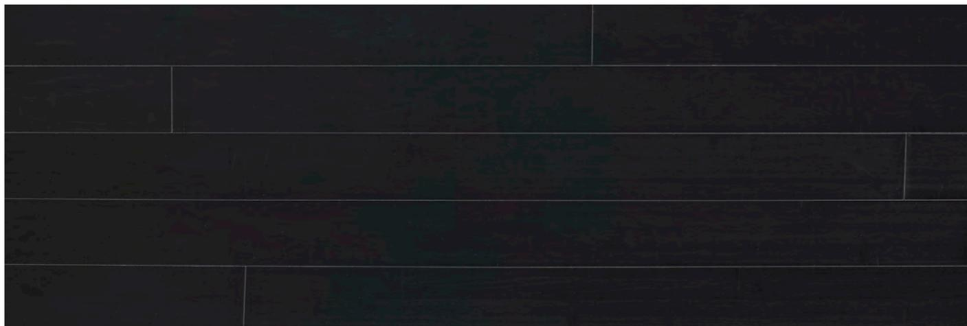
The floor is primed with a black toned water based lacquer system followed by several coats of UV-light curing lacquer. Top finished with an ultra matt two-component polyurethane lacquer.
