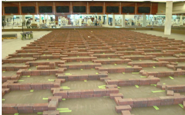
10 mm Sport Tile Installation utilizing 2 bricks head seam 1 brick side seam
